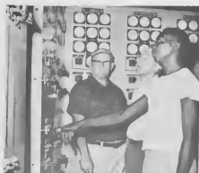
IN ONE of the moves preparatory to switching in the Balashi electrical source at Powerhouse No. 1, F. N. Clark turned on a synchroscope plug. Watchmen are W. R. Moore and C. R. Osborn, both of Utilities.
